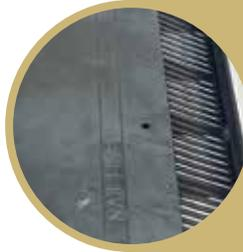
**Pre-drilled nail holes for proper fastening of vent**
